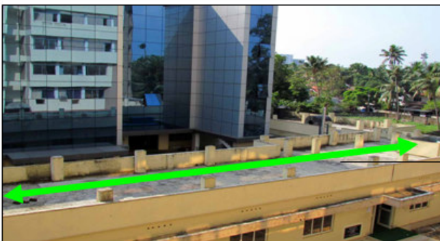
Front view of the construction site on top of canteen building
