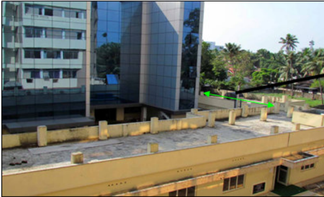
Front view of the construction site
