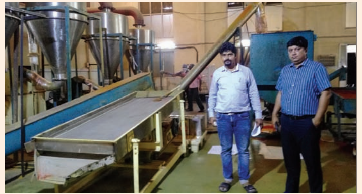
Inspection of Spice Processing Unit at Ahmedabad, Gujarat
